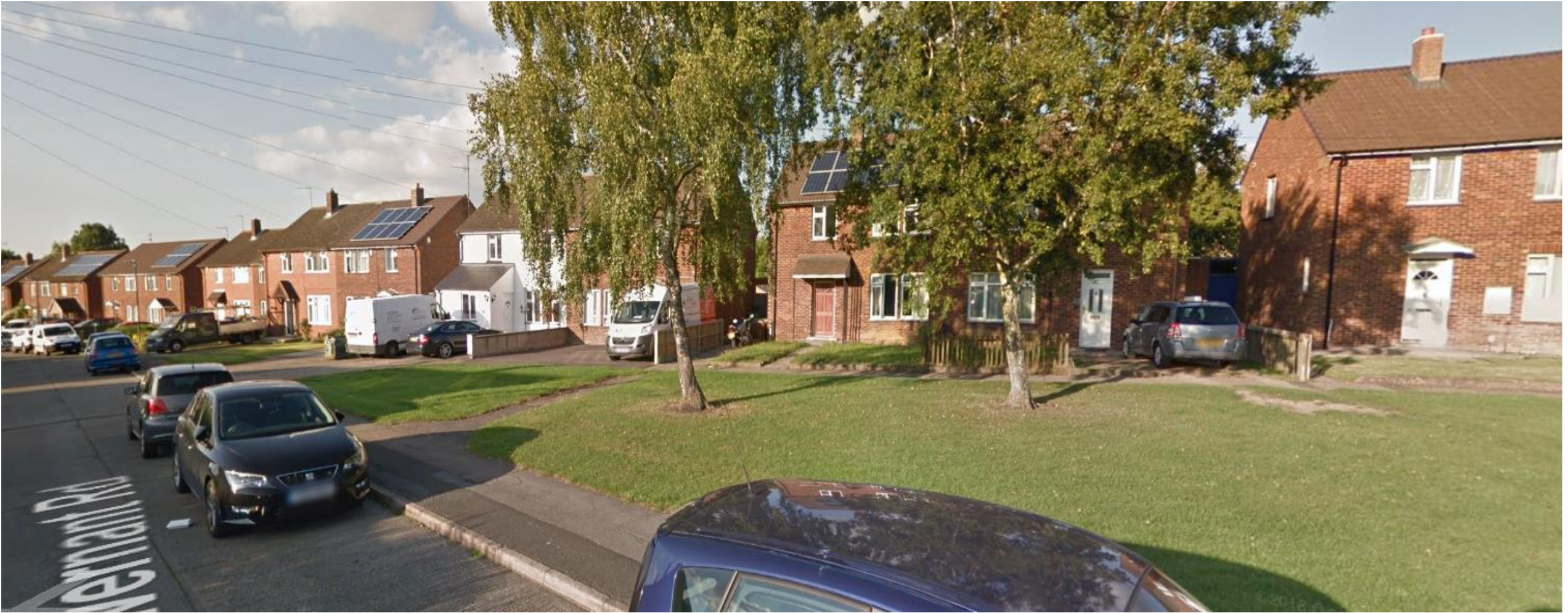
Application site properties in Gwernant Road
